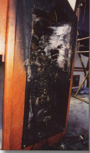
Adding a larger circuit breaker to a distribution panel without also upgrading the wiring can cause the wire to overheat inside the panel and ignite.
